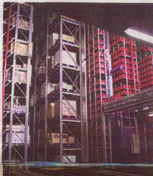
THE HIGH BAY warehouse is fully automated.
